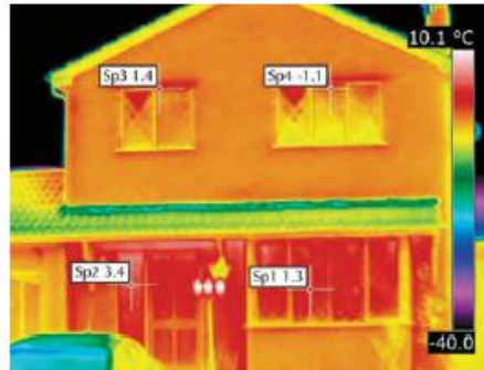
BEFORE and AFTER: The above thermal images clearly demonstrate the advantages of installing new energy efficient windows. The heat loss temperature of the living room window is 1.3°C before and -4.5°C after the new windows were fitted - a significant reduction.
