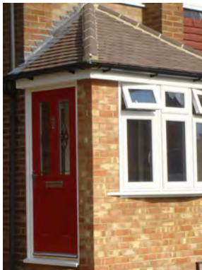
Special Internal Corner Roof
